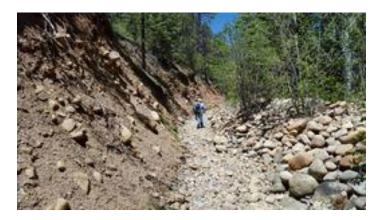
Memphis District engineers survey a section of the Chamisal Acequia to design a solution that will help keep the acequia flowing and clear of loose cobbles and boulders.
