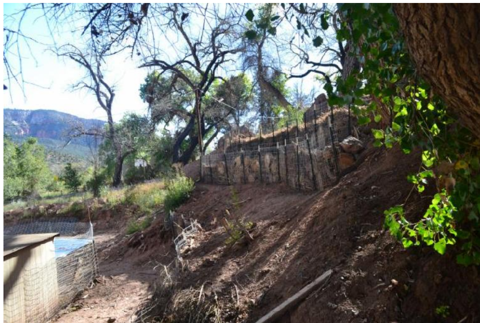
West Sandoval Ditch Bank Stabilization- Photo taken by Juanita Revak
