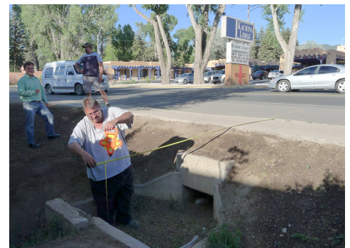
Bobby Jaramillo makes measurements on a culvert of a lateral of the Acequia del Pueblo. Mathew Foster, left, and Charles Chacon, right, stand in background. This lateral has hundreds of feet in culverts under sidewalks and parking lots that are clogged, too small, or otherwise impacted by development along Paseo del Pueblo Norte where the water cannot currently flow. The Task Force is charged to identify these problems for the Town and make recommendations for their correction. Photo by Miguel Santistevan.
